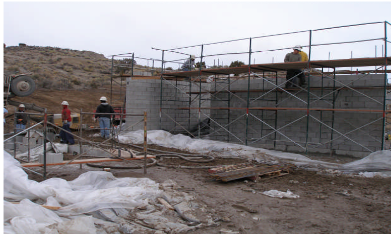
Walls going up that Elko center
