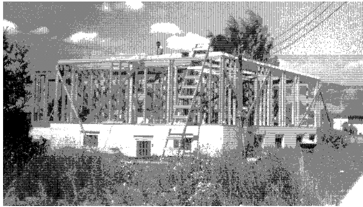
John's house under construction in 1965
