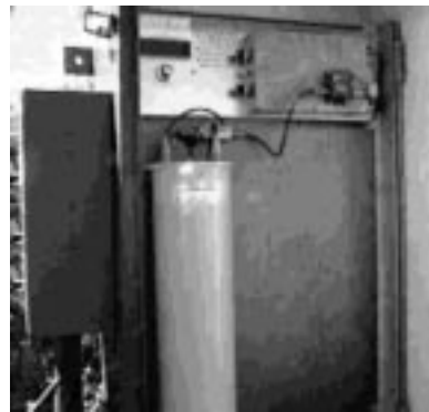
Inside the receive cabinet, there is a receive cavity, the vertically-oriented cylinder in the picture
