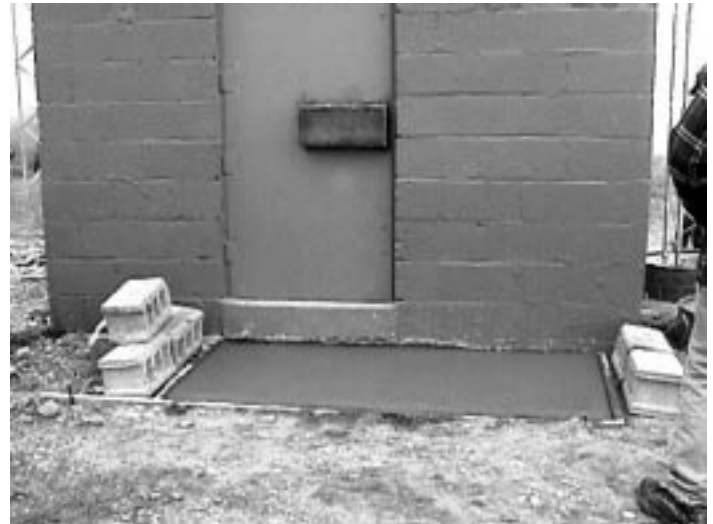
The lock box which now awaits a coat of paint.
