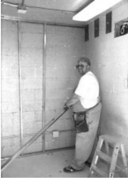
Gregg Smith, KD7APW, starts the inside framing with the metal studs.
