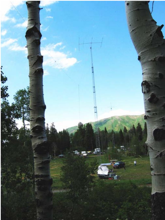
The tall (foreground) tower is the 100-foot unit belonging to W7PS. The one just to the right is UARC's own new 85-foot tower.
