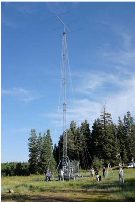
The 85-foot tower dominates the site
