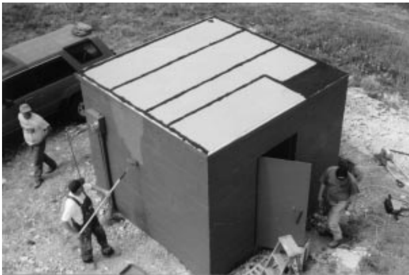
Looking down on the UARC building one can see the section where John ran short of roll roofing - since corrected but leaking still.
