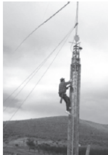
Ropes, pulleys and Mark - Ready to raise the beam.
